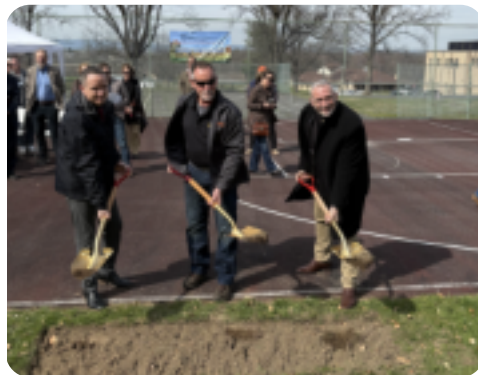
Pictured from left to right: Deputy CEO Nick Hill, Lancaster Asphalt Owner & President Wesley Powers, and Bethany President & CEO Dr. Joseph Birli take part in the commemorative groundbreaking to celebrate the start of construction.
